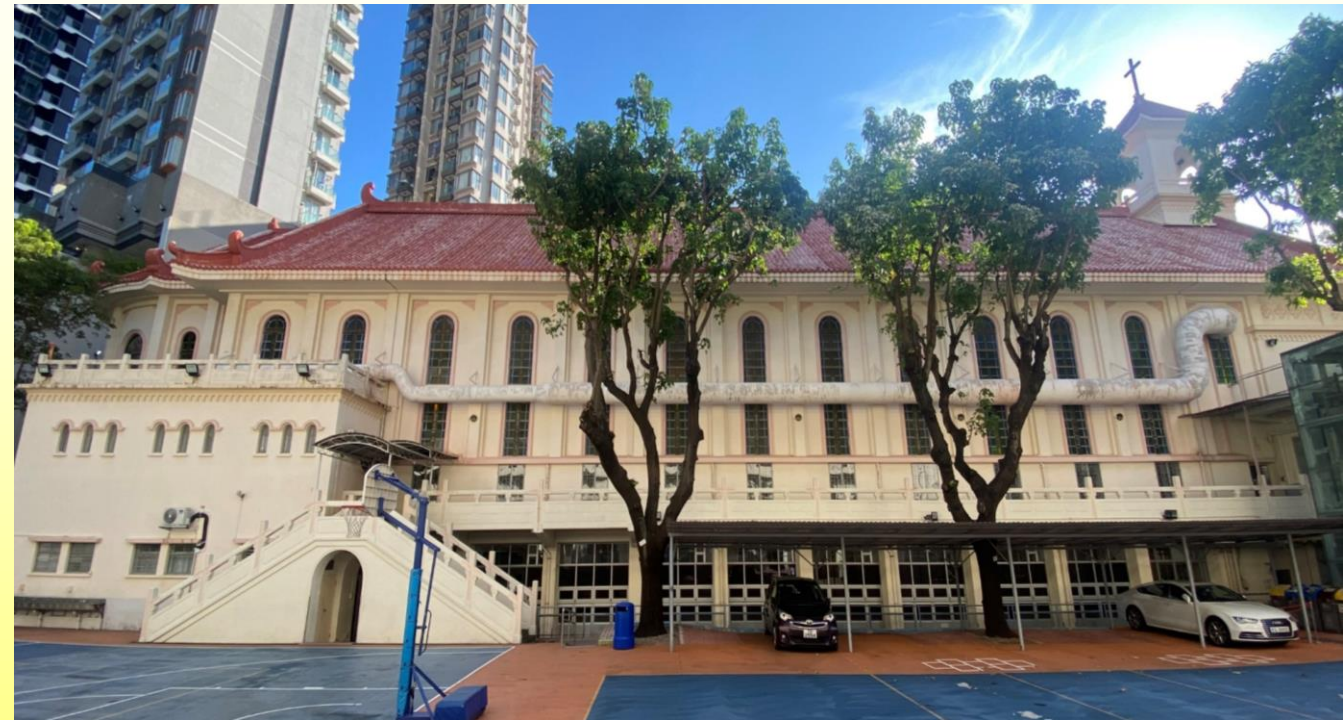
面向學校球場的側立面 Side elevation facing school's ball court
